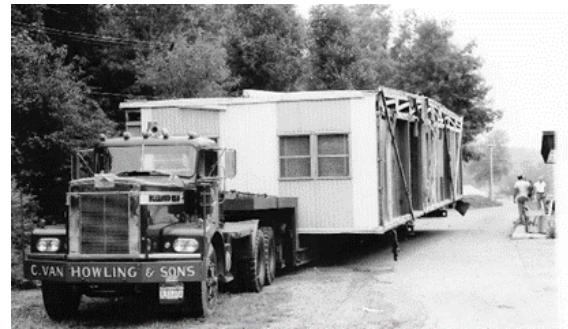
Transportation of the construction trailers to the municipal complex. They were used by AT&T during construction at one of their sites in central New Jersey. Circa 1975.
