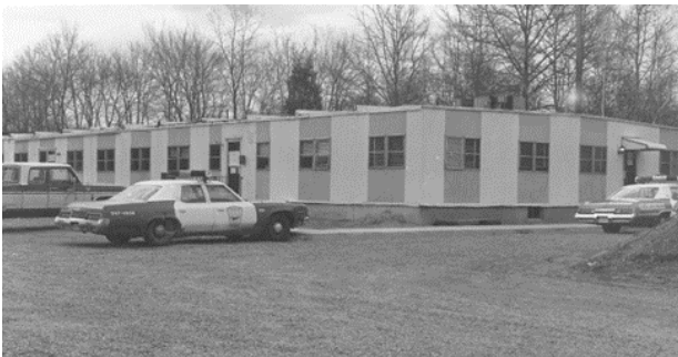
Municipal Building shortly after assembly. The existing structure is comprised of used construction trailers. Later, a shed roof and façade were installed. Circa 1975.
